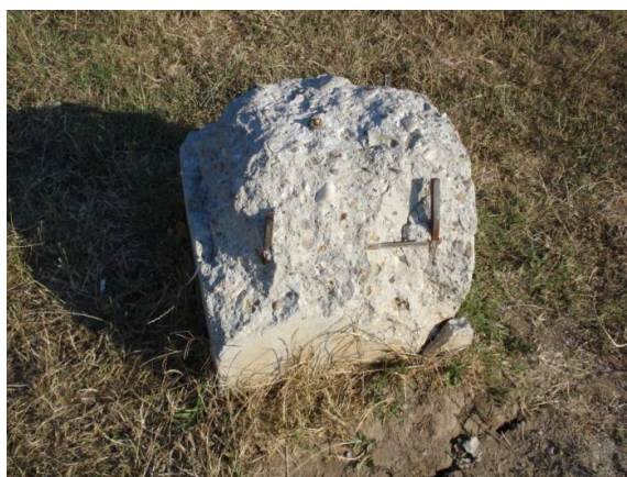
Fig. 3.3.10. Examples of destruction of network benchmarks.
