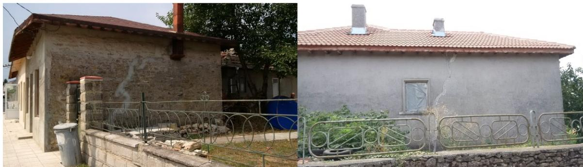
Fig. 20 – Oblique cracks, considered to be due to active faulting, observed on houses walls in Shabla (left) and Ezerets (right) localities.
